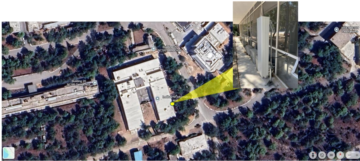
Figure 66 - The new antenna shown in situ on the NCSR Campus
