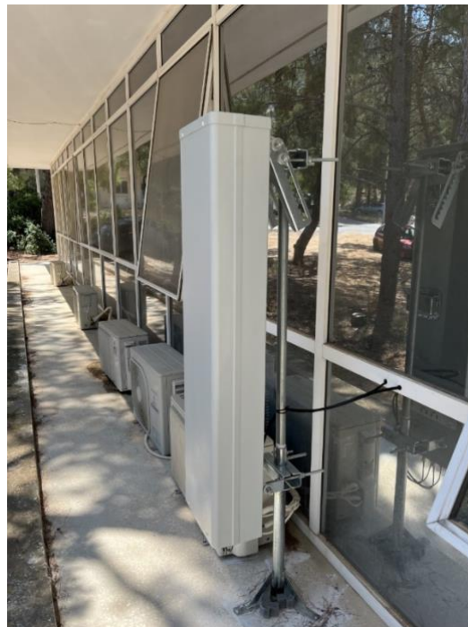
Figure 9: Amarisoft RAN equipment for signal quality metrics acquisition at NCSR Campus.
